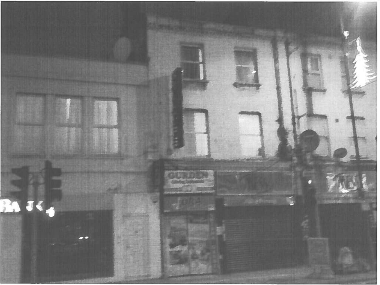
(Showing external entrance of premises as seen from Green Lanes)
